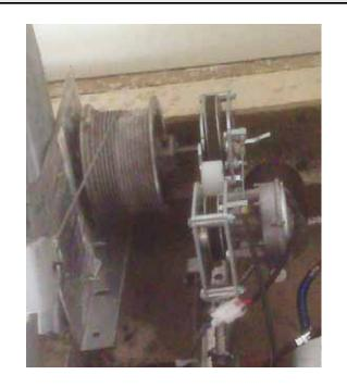
Commercial Operator Front Mount Low Head Room Mounting
